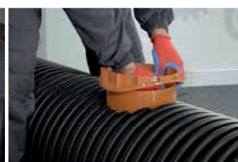
8. setting the spacer ring
