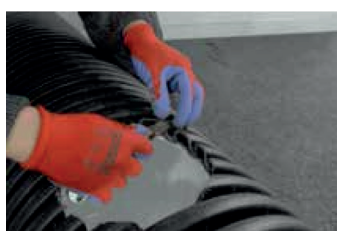
5. Cleaning chips and forming a clear hole
