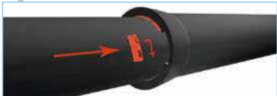
6. Connecting the pipes and inserting stoppers
